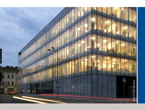
semi-transparent effect and special shine to OKATECH insulating glass with metal inserts from OKALUX. The functional glass softly diffuses the daylight into the interior while protecting it from sun and glare. OKATECHS' large range of different metal wire mesh, expanded metal and perforated sheet make it the perfect choice for a myriad of individual design possibilities. Kuba & Pilař Architects chose a variant with ano-
